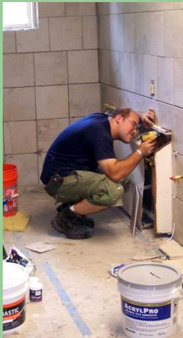
PHOTO TAKEN DURING 2015 USA RENOVATIONS WEEK
