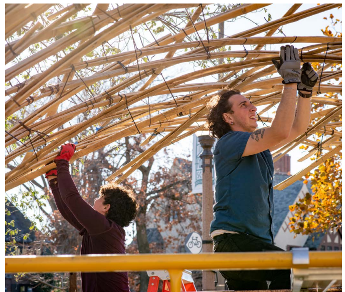
Student volunteers worked with Assistant Professor Wyly Brown and visiting bamboo expert Hans Hernandez to construct a bamboo shelter for the new Peace Park site in north St. Louis. Photo: Carol Green.
