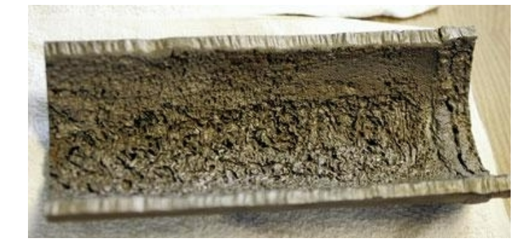
"Corroded Section of Prudhoe Bay Oil Field Pipeline." The Denver Post, The Associated Press, 6 Aug. 2006. www.denverpost.com/2006/08/06/bp-closing-alaska-oil-operation-indefinitely/.
