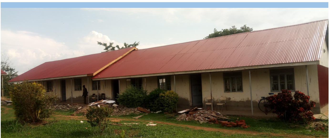
Lecture Room at final stage of completion
